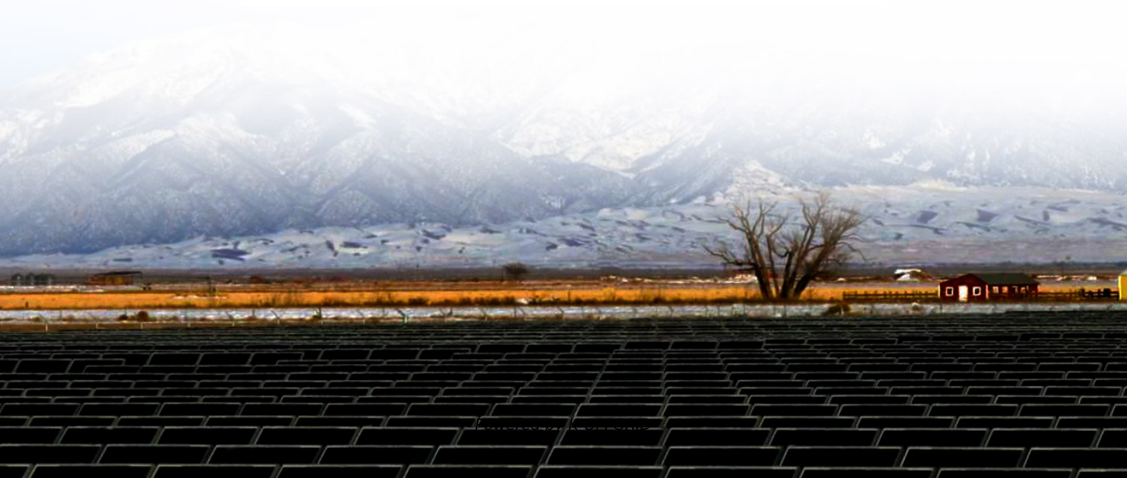
200kWh Battery Cluster
